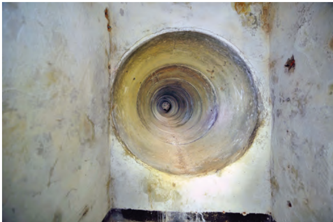
The emergency escape tunnel. Photo Chris Warren
